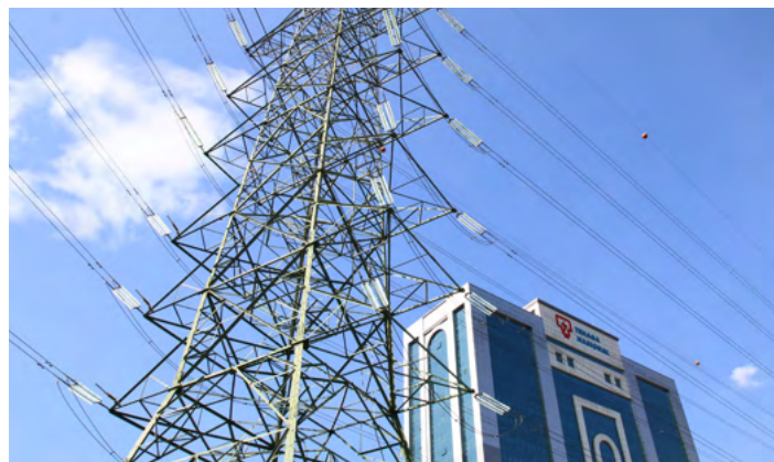
► Tenaga Nasional's transmission tower
